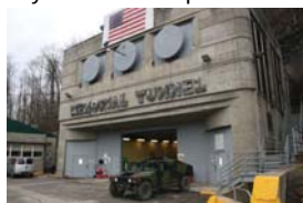
Entrance of the Memorial tunnel
